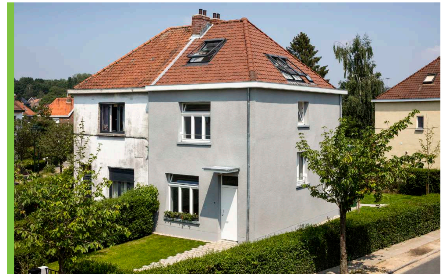
RenovActive, Belgium. Photo: Adam Mørk.
